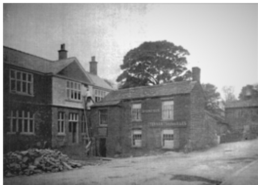
[1904 Building and demolition RA]
