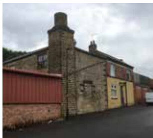
[High House Brewery Chimney 2019 DP]
