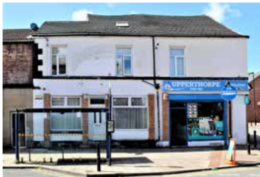
[The Upperthorpe Hotel DP]
