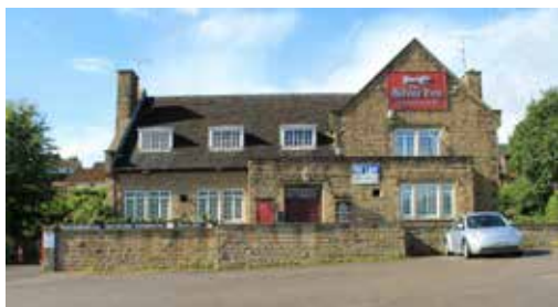
[The Silver Fox: to be demolished DP]
