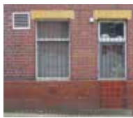
[Original entrance for off-sales DP]
