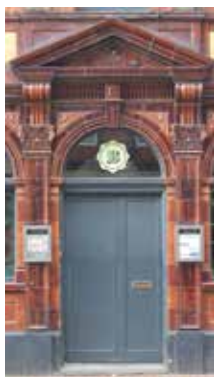
[tilework around the door DP]
