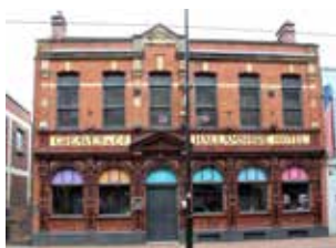
[Ornate tilework DP]
